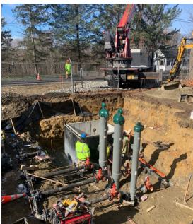
Town of Bennington, VT Municipal Line Extension for PFOA Remediation
